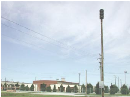
Base alert warning system.
