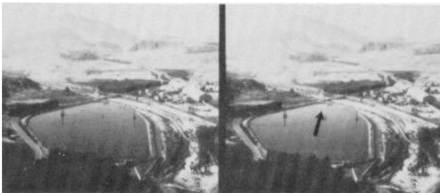
Figure 2-17. Overhead Bucket Conveyors over Pond.
