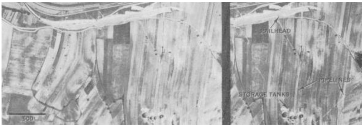
Figure 2-32. Storage Tanks and Pipelines.
