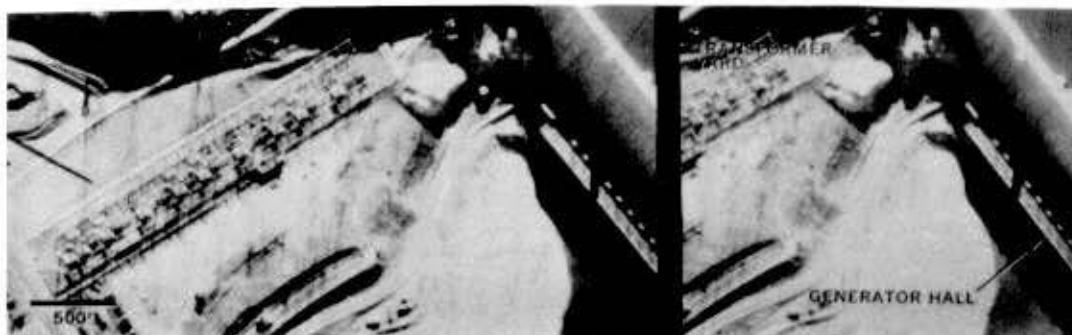
Figure A-53. Transformer Yard.
