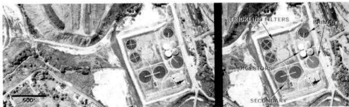
Figure A-32. Primary and Secondary Sedimentation Tanks.
