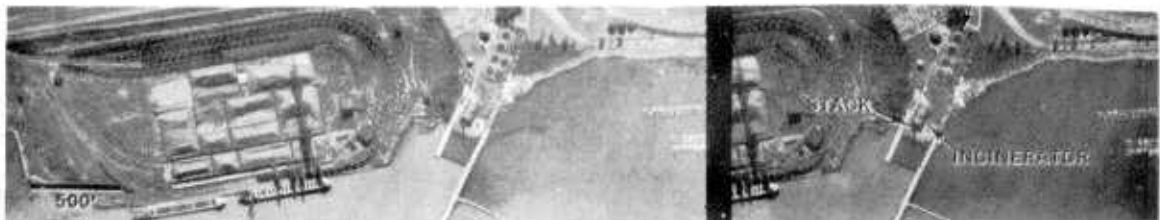
Figure A-2. Stack for Sewage Incinerator.
