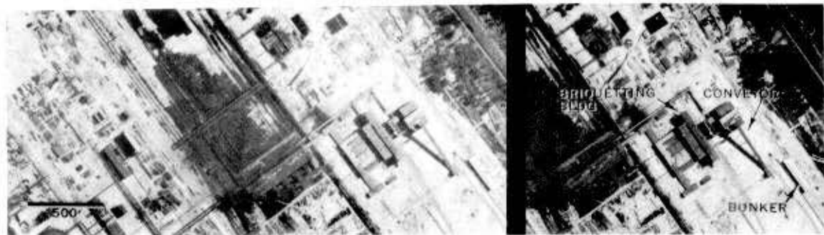
Figure A-46. Coal Conveyor.
