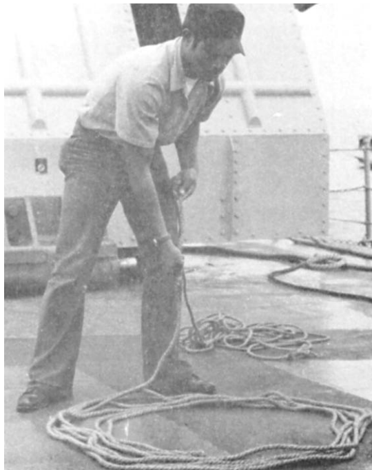
Figure 3-3.—Coiling down a line.
