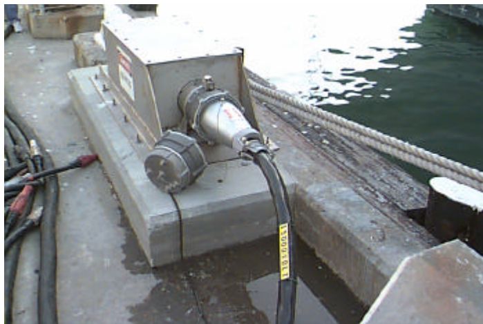
Figure 12-1 Electrical connection outlet assembly with a 15-kV receptacle
