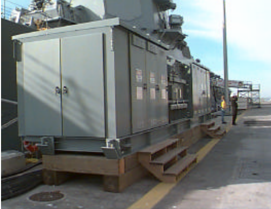
Figure 12-2 A skid-mounted substation
