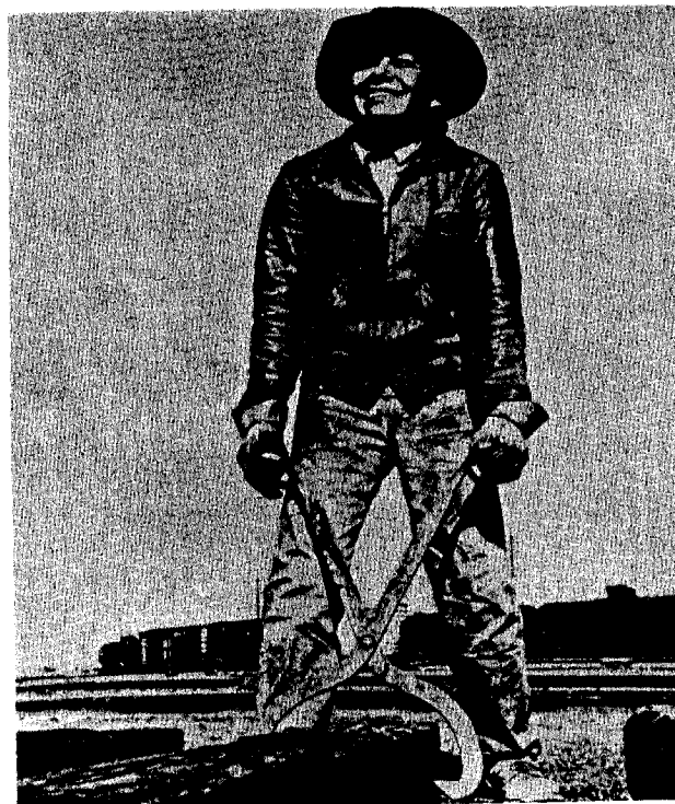
Figure 3-16. Handling treated wood ties.
