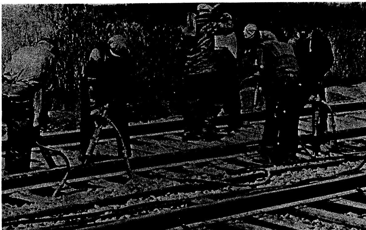
Figure 3-7. Manually tamping ballast with compressed air tools.
