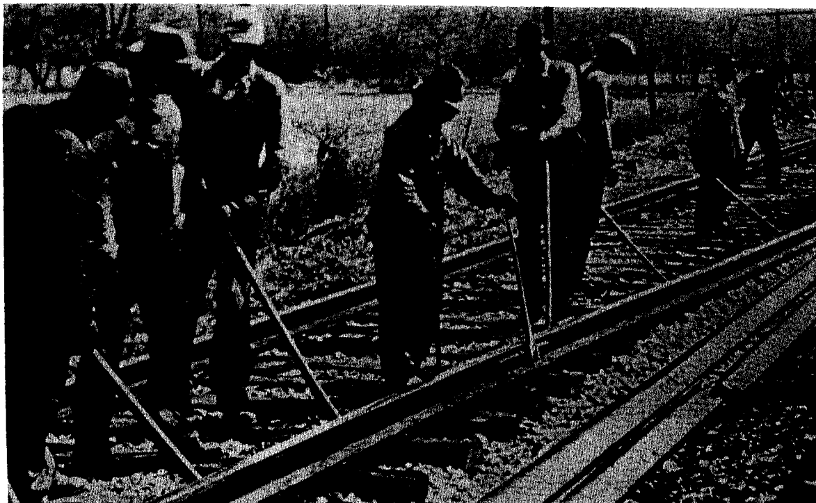
Figure 3-36. Rail being lined out.
