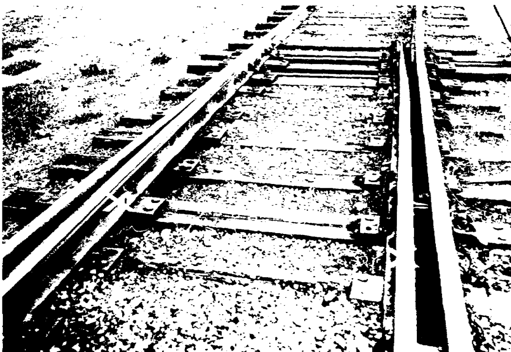
Figure 2.5. Split Switch Thrown for Turnout Movement.
