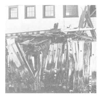
Figure 7-24.—Broken wood piles.
