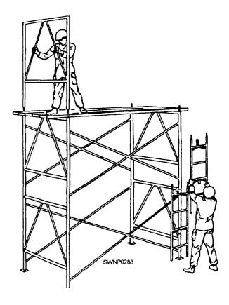
Figure 6-41.—Assembling prefabricated independent scaffolding.
