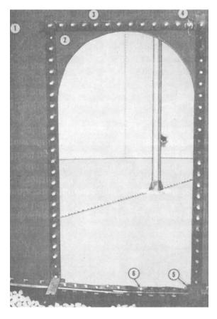
Figure 9-24.—Bolts installed at cleanout opening.
