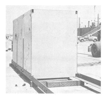
Figure 10-22.—P1 pontoons on assembly angles
