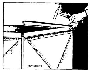
Figure 2-96.—Placing S slips for S-and-drive connection.
