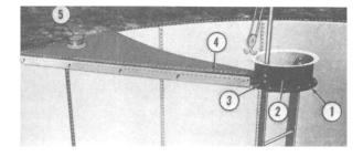
Figure 9-17.—First deck plate installed.
