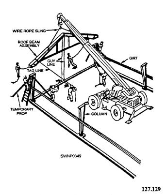
Figure 8-6.—Using power equipment.
