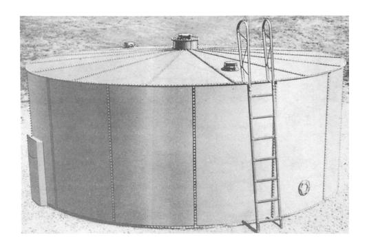
Figure 9-5.—500-barrel capacity vertical, bolted steel tank assembled.
