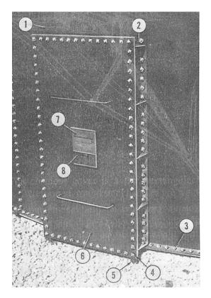
Figure 9-25.—Cleanout cover installed.
