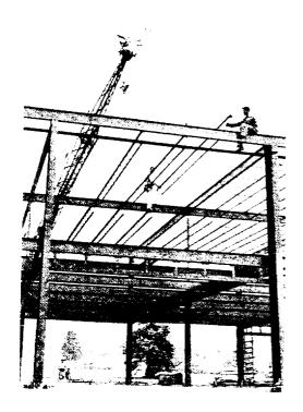
Figure 3-20.—Installing bar Joists girder to girder.
