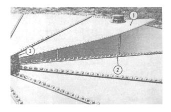
Figure 9-20.—Installing last deck plate.
