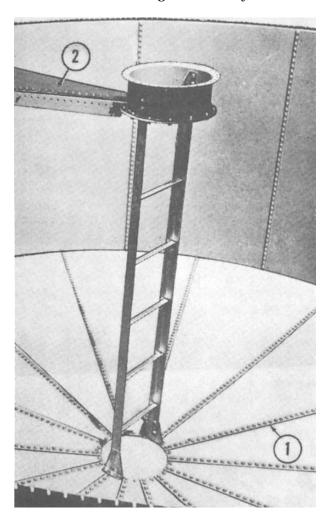
Figure 9-18.—Center support ladder installed.
