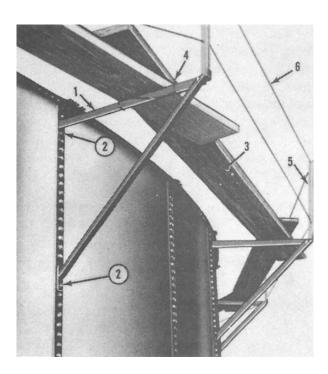
Figure 9-13.—I.ocation of the scaffold around the top chime of the staves.
