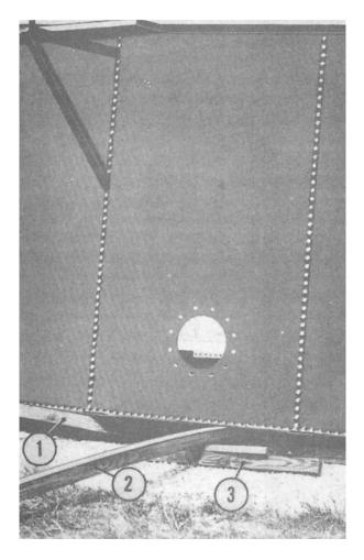
Figure 9-14.—Removing the timber blocking.
