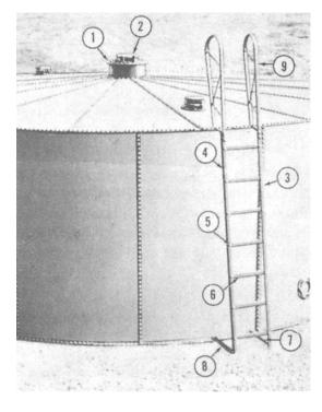
Figure 9-21.—Outside ladder installed.
