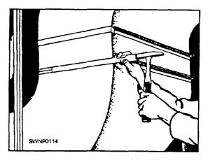
Figure 2-97.—Inserting drive slips.
